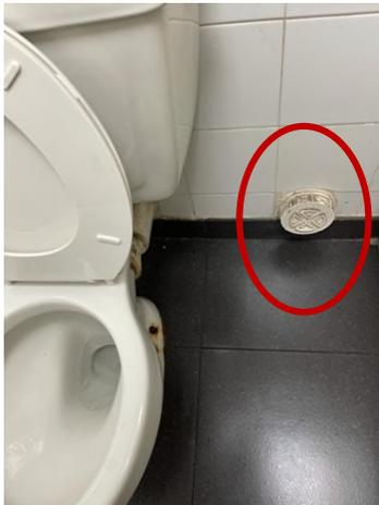
make cleaning difficult and create a breeding ground for germs. Where the pipes change direction, it's important to install rodding eyes to allow for easy cleaning and maintenance in case of blockages.
