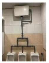
replenished after the previous flush, which may require a couple of minutes or longer.For environmental protection, waterless urinals are an alternative because they don't require the flushing of water; however, frequent inspections are required to
