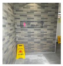
2.4.2 All drainage and water supply pipes connecting to the sanitary appliances should be securely fixed and hidden in walls or floors to prevent dirt from getting trapped between the walls and the pipes. This can
